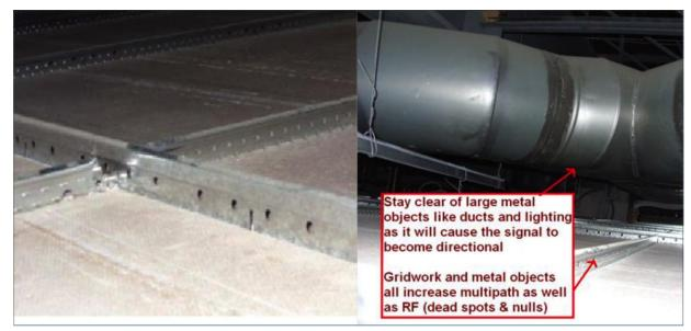
Installing the AP above ceiling tiles: pick an area clear of obstructions, avoid ceiling clutter
