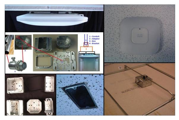
Mounting an AP onto an electrical conduit box (ceiling T-bar or conduit)
