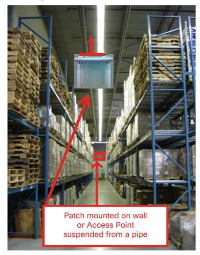
AP Placement in warehouse environment (External dipole "e" series or internal antenna "i" series version could be used)
